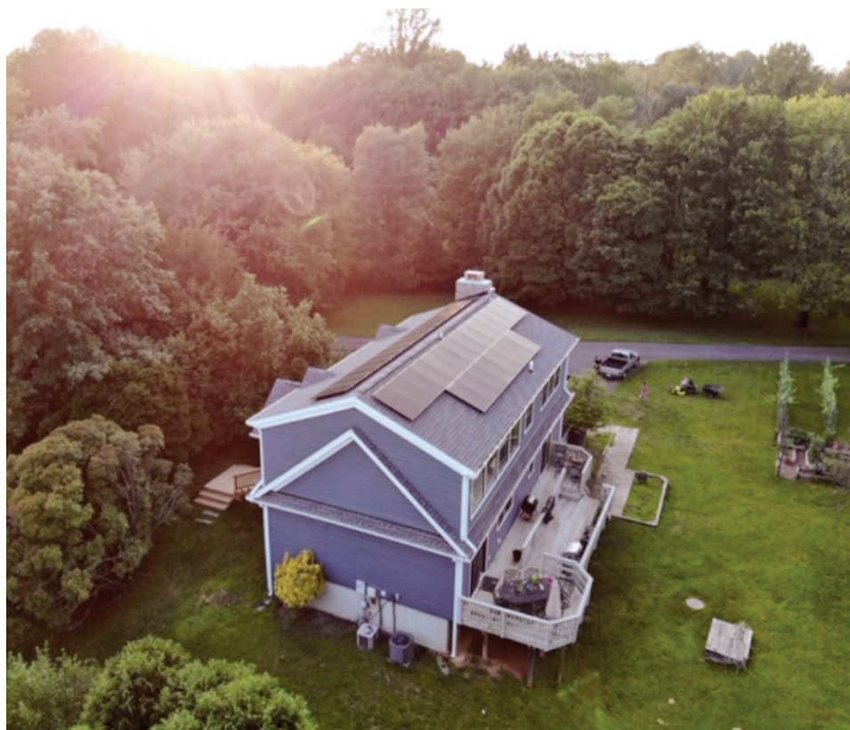
Wen Family home, pictured from above, showing off their solar panels.
